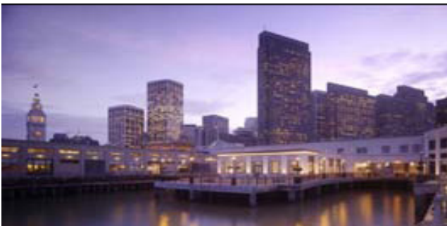
Pier 1 ½ after revitalization
