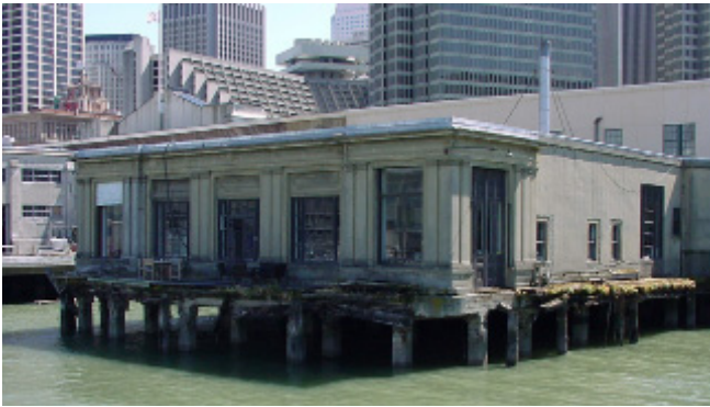
Pier 1 ½ before revitalization
